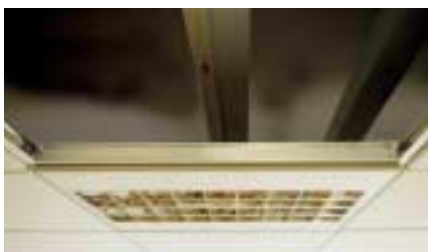
Downward demountability provides easy access to the ceiling void
