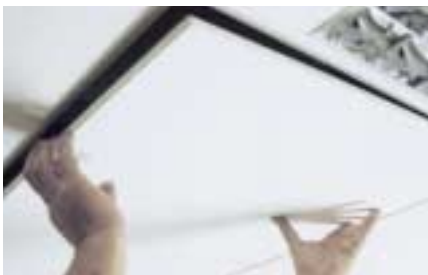
Tiles can be removed from below without the aid of a tool
